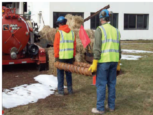
Reenactment of Workers Carrying Augers
