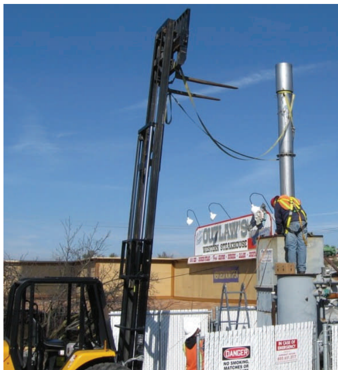
Subcontractor Maco Industries, working at heights Atascadero, CA
